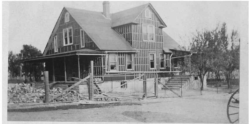
Gus Pinter farm house under construction, date unknown (Half mile north of Ladd)
