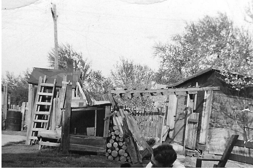
Filippini outdoor “facilities”, Ladd, IL
